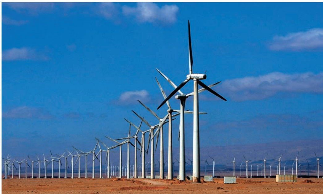
■ Giant wind turbines generate electricity at the Zafarana Wind Farm along the Red Sea Coast, Egypt. Egypt plans to meet 12 per cent of its energy needs with wind power by 2020
